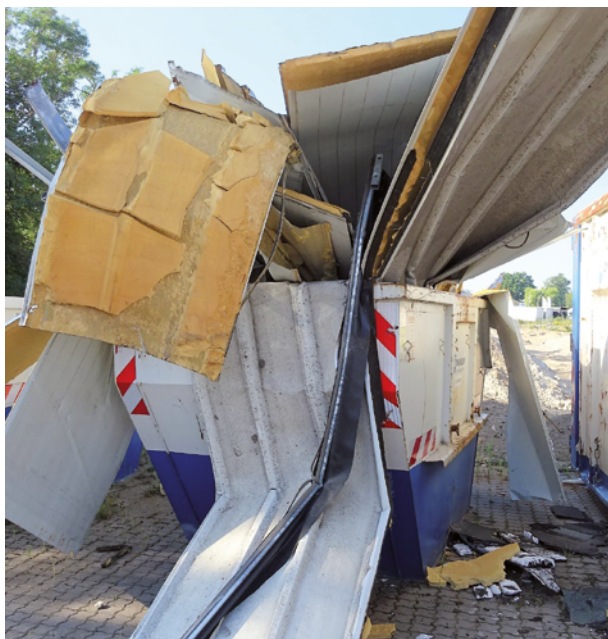
Mixed construction waste unsuitable for high-quality recycling
